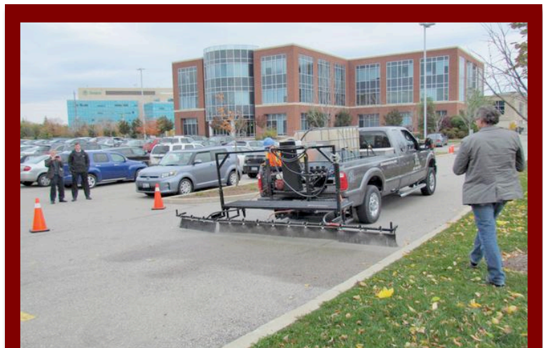
Soy sprouts new industry - Agriculture industry members watched a demonstration of a new agricultural oil seal and preservation agent made by a combination of soybean oil and non-petroleum polymers, offering an environmentally-friendly and cost effective way to maintain asphalt surfaces. photo by Kelly Waterhouse
