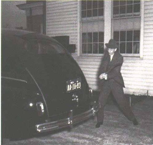
Henry Ford testing the impact strength of a soy flour composite decklid, 1940.
